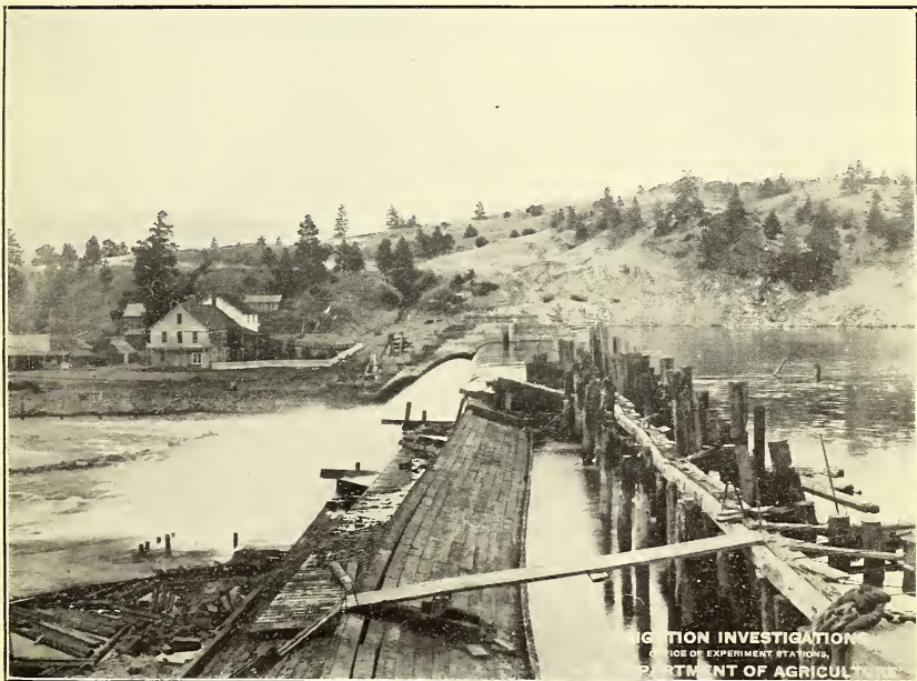
FIG. 2.—CANYON FERRY DAM, BEFORE RECONSTRUCTION.
